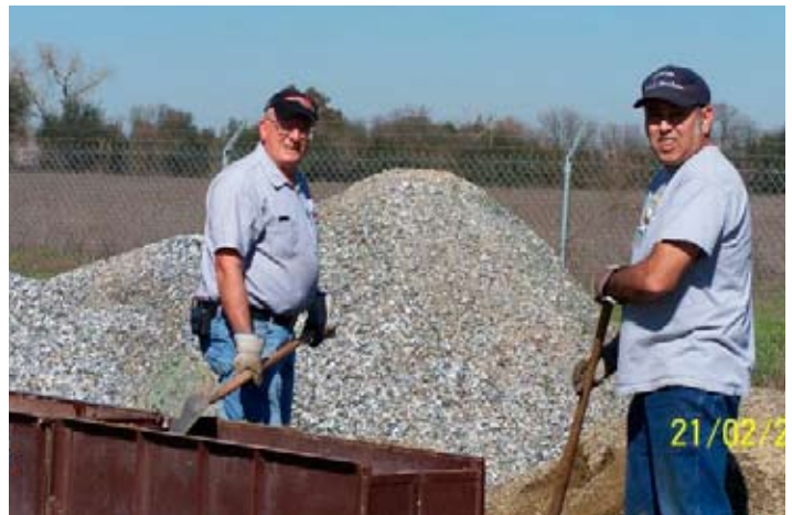
Pete Arney and Darrell Gomes (doing multiple jobs on work days) loading the gravel car after re-ballasting the ties. This is a never ending task that always needs good help to keep the track in good shape. Thanks !!!
