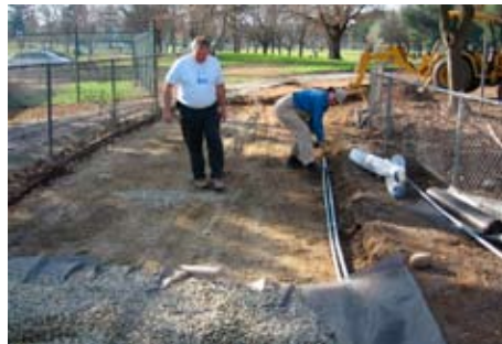
Bill, Lee adding electrical & signals lines
