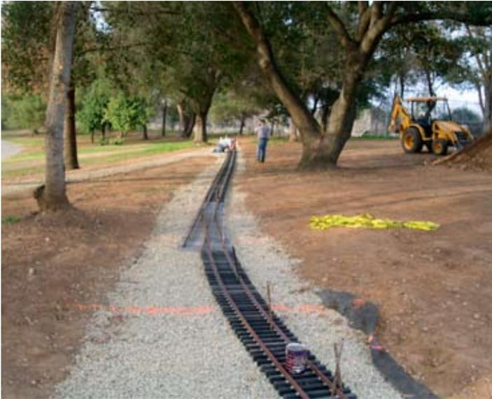
Rail being added to ties for new station track.
