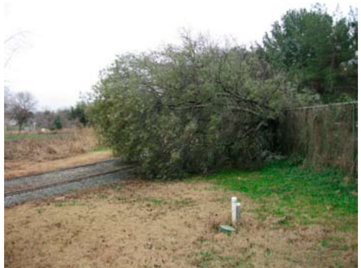
Recent wind damage, tree crossed over the Sugar Pine track, over the fence, and onto mainline.
