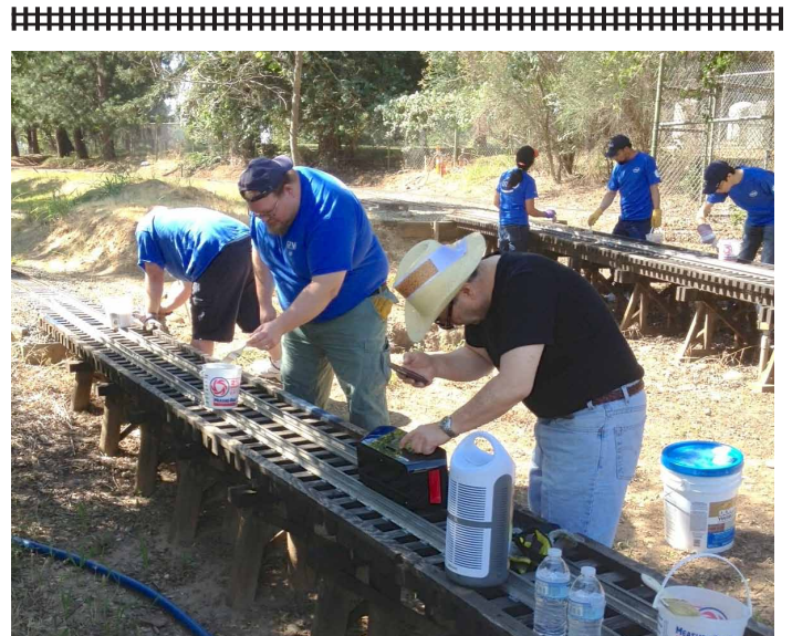
Intel crew volunteers providing needed maintenance on our trestle.
