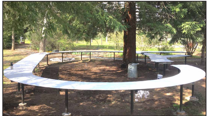
Phase one table progress
