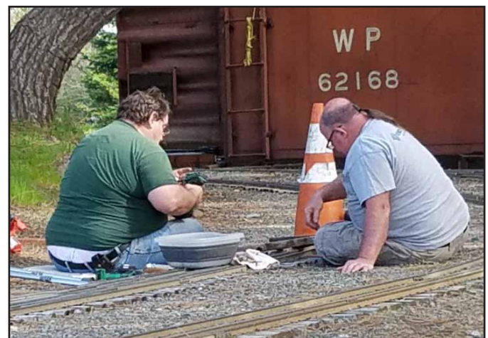
Dennis and Craig working on station switch.
