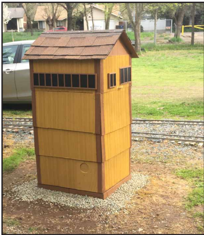
Touch up of Mercer tower
