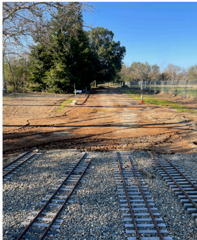
Now ready for roadbed
