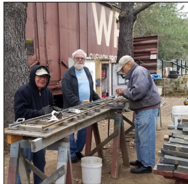
Paul Skidmore, David Cladianos, Butch Floyd continue working on building track.
