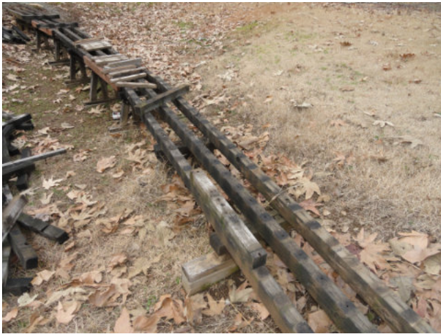
View of Trestle west of Reverso switch.
