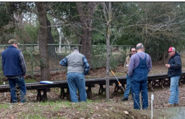
Steve Milward track superintendent and his bridge replacement volunteers.
