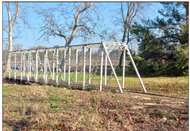
Rob & Andy removed tree that fell down on "Tin Man Bridge"
