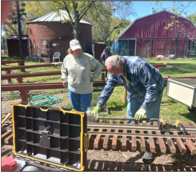
Steve Milward replacing wood ties on lead tracks with Stephanie Huntingdale watchful eye.
