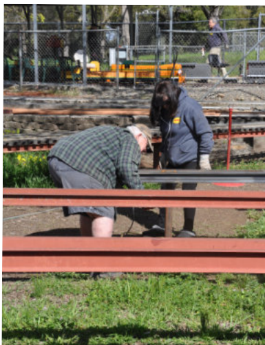
Keith & Gloria Berry working on added steaming bays.
