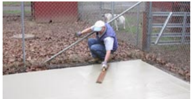
Pete Arney - putting finishing touches on new pad for storage shed. Just one of the many projects that Pete completed in 2004 for SVLS . Thanks Pete for your dedication to make the SVLS facility a great place.
