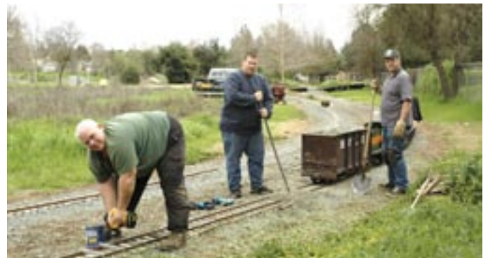
Keith, Gordan, Richard, and Pete (elsewhere) installing new steel rail.
