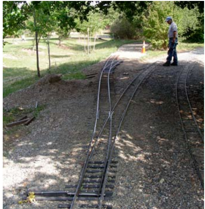
Progress is being made on building the new yard at Midway.
