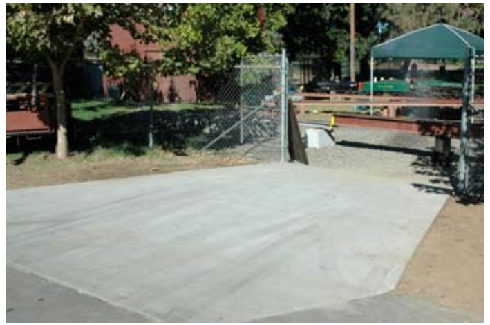
The new concrete pad which raised the loading area by 6 inches made the process much easier.
