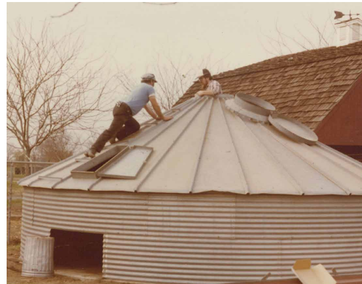
Installing club roundhouse that was donated by Rod Danley. Edwin Yungling is climbing the roof panel.
